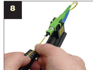
**8** Open the activator tab and insert fiber into the connector. Refer to point D for fiber insertion depth.
