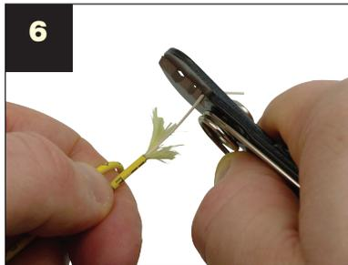
**6** Wrap fiber cable around finger, then strip off buffer to point C\*
