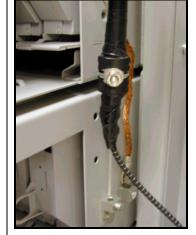
15. Insert the Strength Member of the Cable into the Ground Lug.
